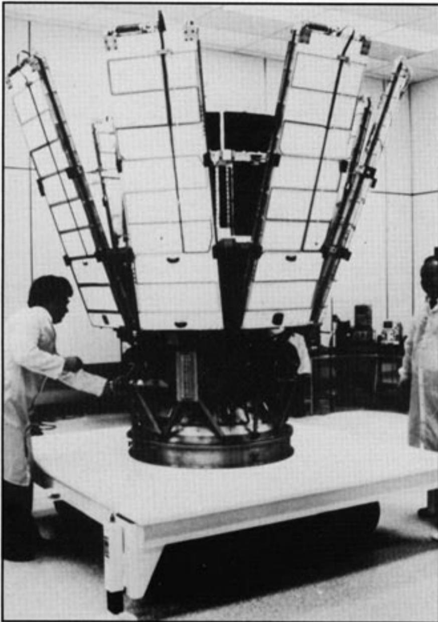
Fig. 11 Geosat-A spacecraft prior to being mated to the OIS upper-stage. (DOD Still Media Depository)
