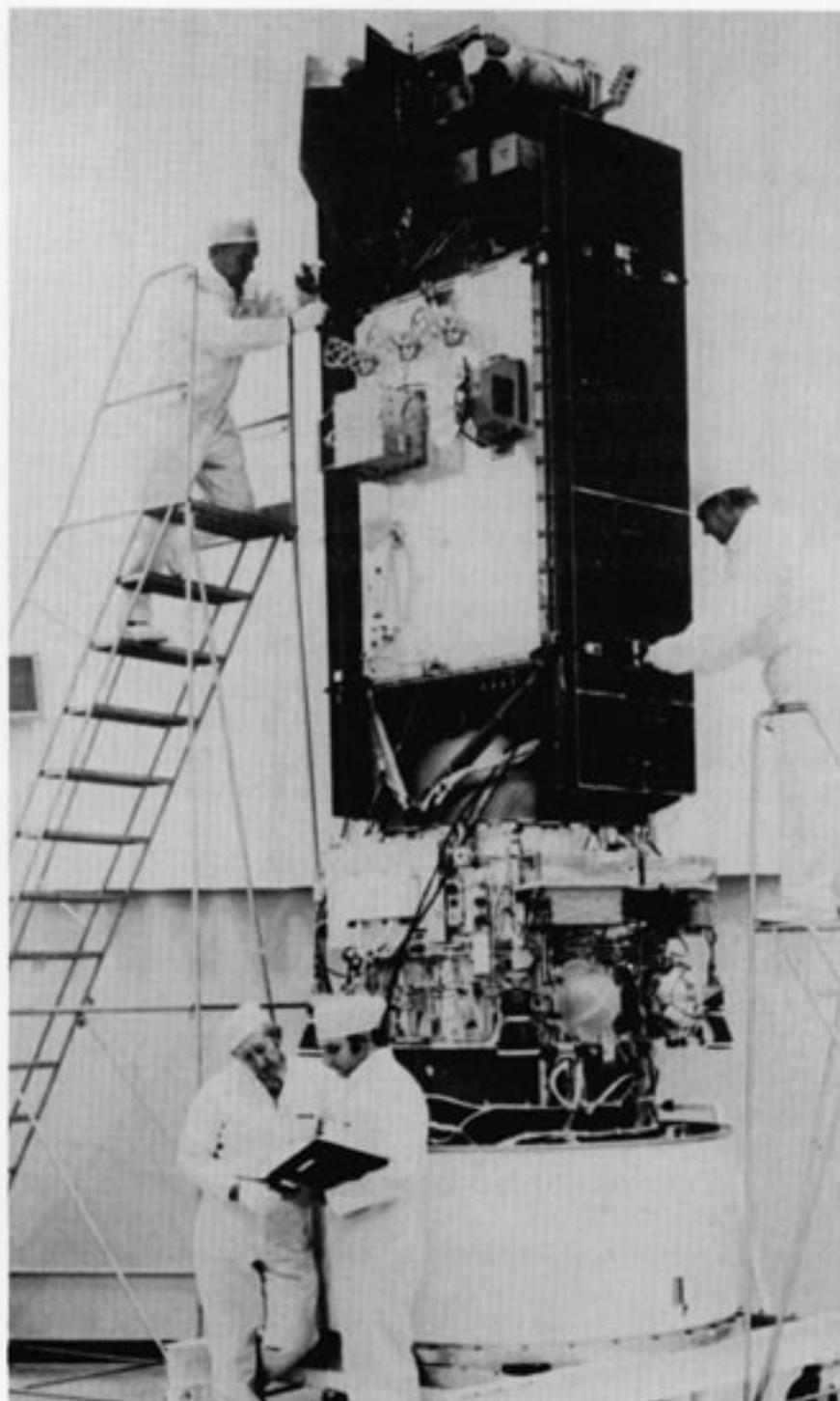
Fig. 10 The solid motor of the ISS upper stage can be glimpsed in the mid-section of this Block 5D-2 DMSP weather satellite. (RCA Astro-Electronics)
